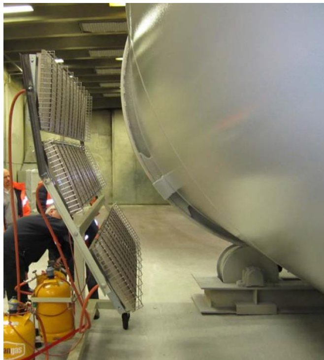
Figure 3: Setting up the IR heating unit
